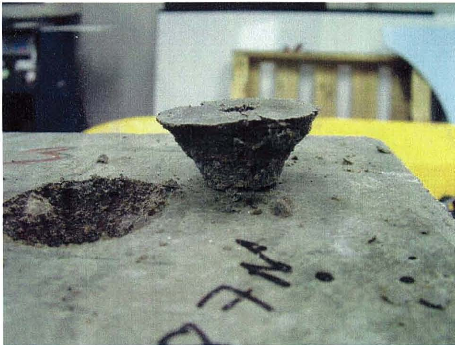
Figure 7 – Typical Failure Surface of Pullout Test (Extracted Cone)
