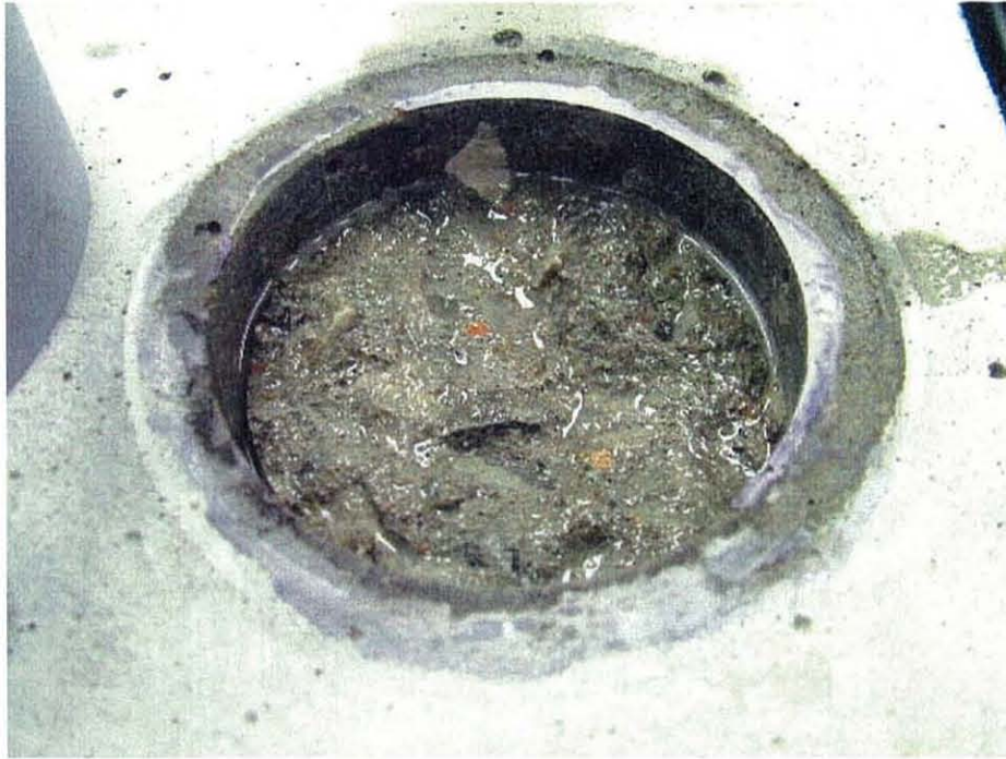
Figure 12 – Typical Failure Surface of Direct Tension Test
