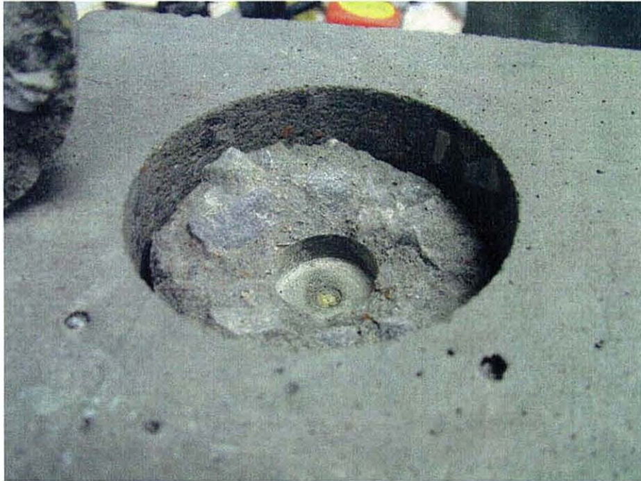
Figure 14 – Typical Failure Surface of Modified Pullout Test
