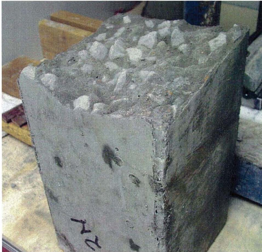
Figure 33 – Example of Coarse-Aggregate Pullout (Beam Tested in Flexure)
