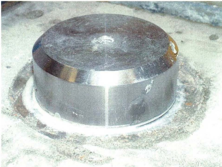
Figure 9 – Steel Disk Adhered to Prepared Concrete Surface Prior to Coring for Direct Tension Test
