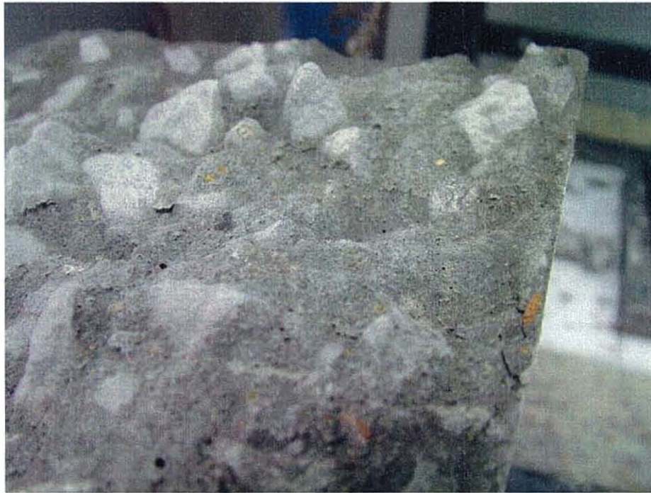
Figure 34 – Close-Up View of Coarse-Aggregate Pullout (Beam Tested in Flexure)
