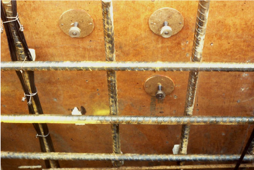
Fig.15. LOK-Test inserts installed in wooden formwork before concrete casting.
