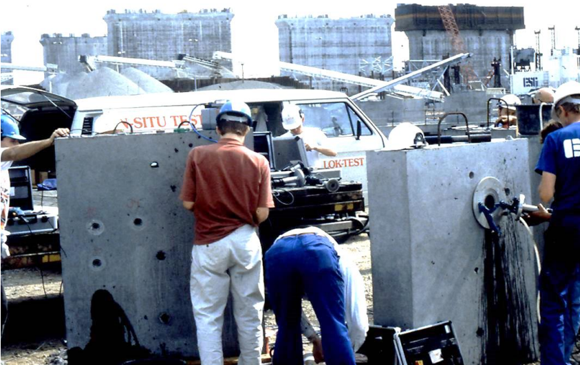
Fig.13. Training of the contractor's technicians on performing LOK-TEST and CAPO-TEST. The training course was completed with an examination and issuing of a diploma.
