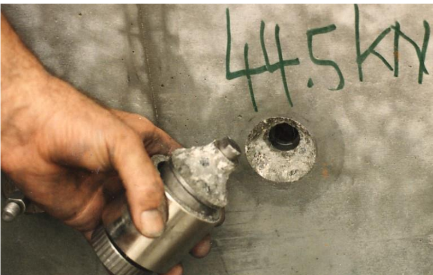
Fig.14. Successfully completed CAPO/LOK-Test of the cover layer of an element.
