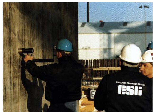
Fig. 7. LOK-test for in-situ strength assessment.
