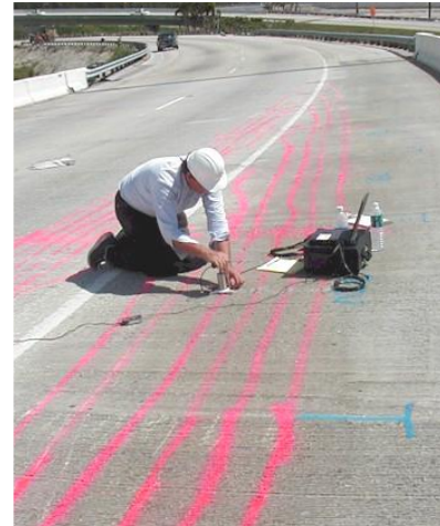
Testing for quality of grout injection in cable ducts
