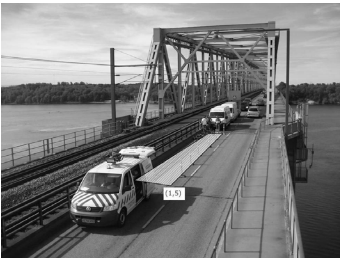
Figure 18. Photo of The old Lillebælt Bridge with one test area in between the cars.
