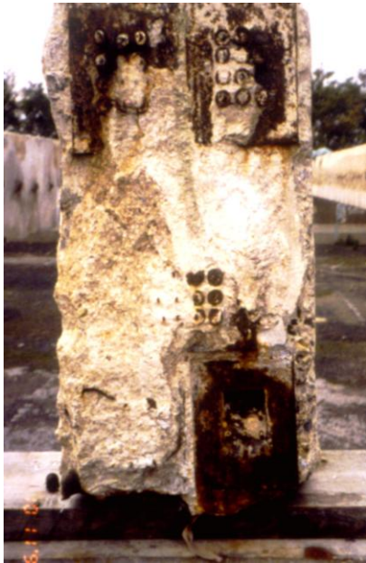
Collapsed beams to be tested for injection of cable ducts, UK
