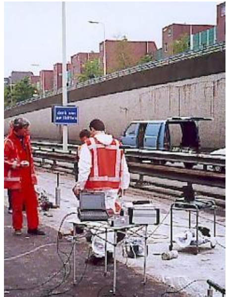
Testing of tightness of highway slab joints, Holland
