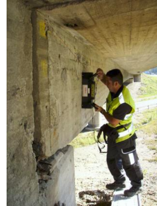
Fig.5. 3D Tomographer testing in progress for cable duct injection
