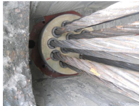
Fig.2. Post-tensioned strands
