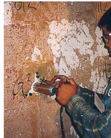
Fig.6. Impact-echo testing of pulp tanks for cold joints
