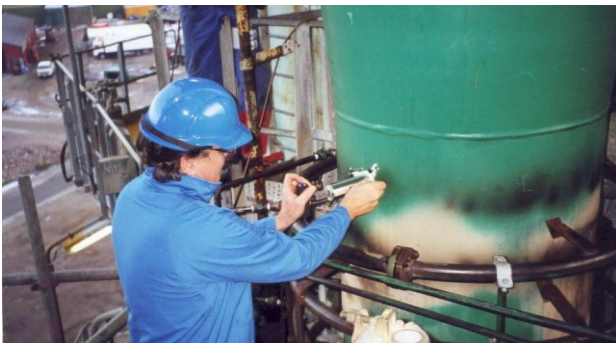
Testing of the thickness of concrete liner inside a steel riser column in a refinery, Sweden
