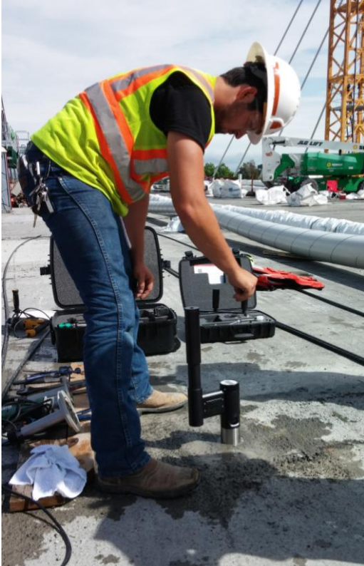
Joints at Ohio River Bridge, Louisville, Kentucky, USA being tested for compressive strength with CAPO-TEST
