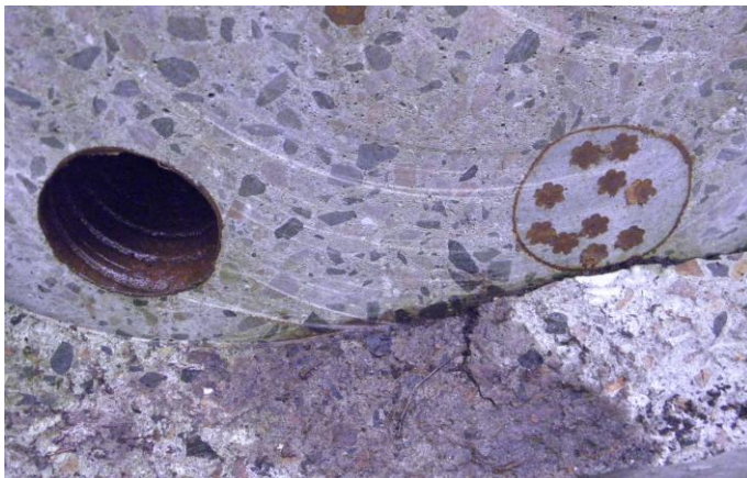
Figure 21. Cut 1 for verification that duct with the 10 strands was fully grouted.
