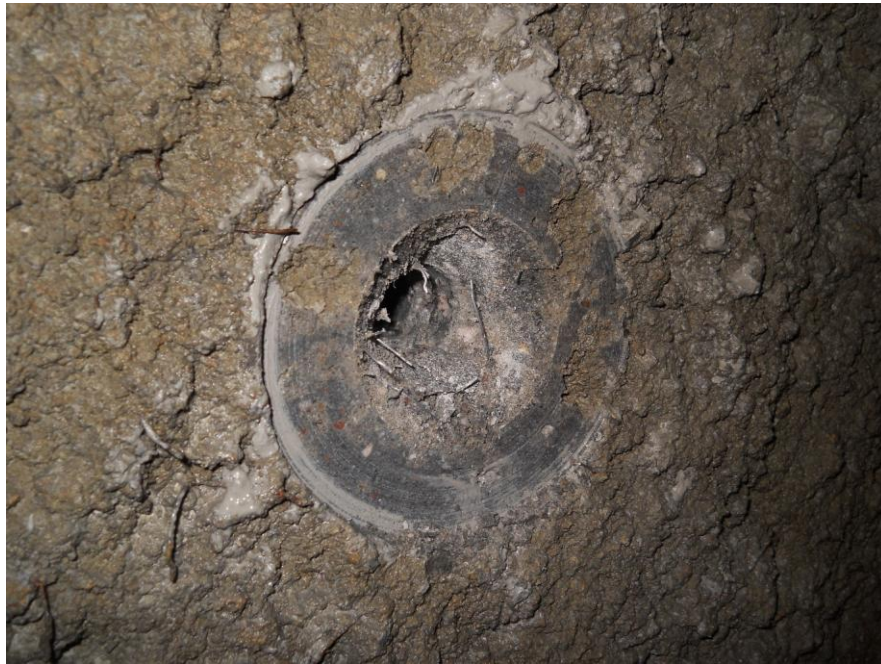
Fig.10 CAPO-TEST failure on shotcrete with steel fibers
