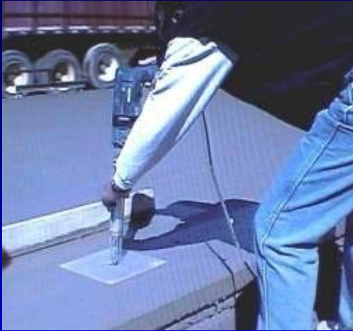
Obtain mortar sample
