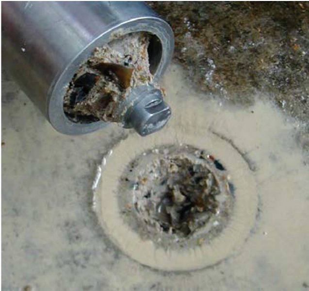
Fig. 3—Example of acceptable CAPO-TEST with complete ring at surface.
