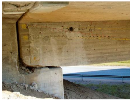
View of web and drilled core
