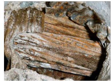
Condition of duct
