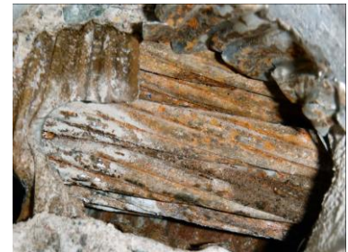
Condition of duct
