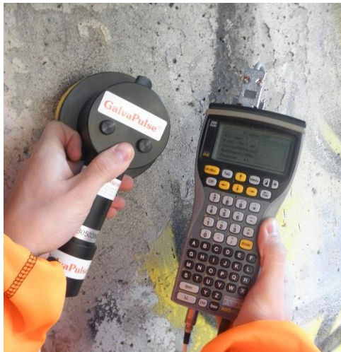
Corrosion activity being evaluated on a bridge wall with the GalvaPulse
