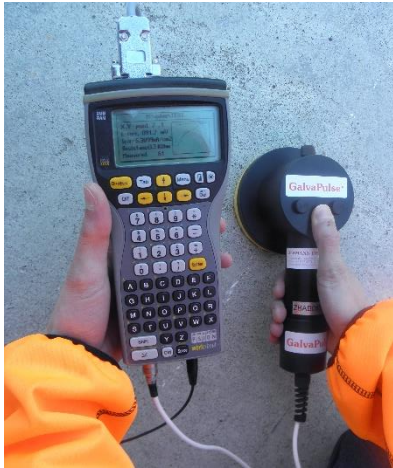
Evaluation of corrosion rate in balcony slab of seaside condominium with the GalvaPulse
