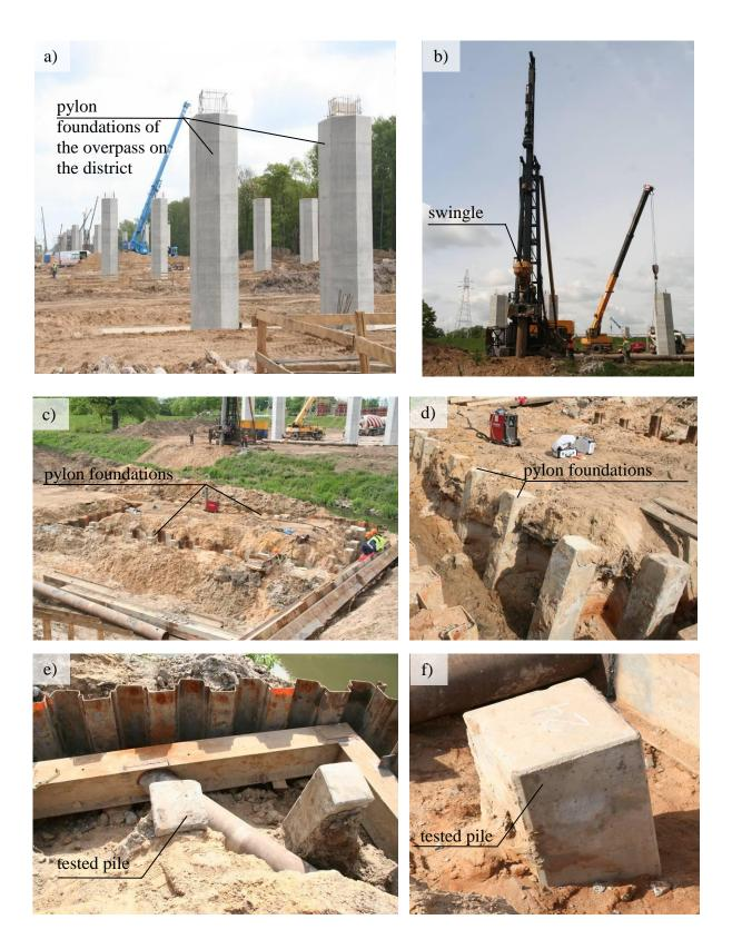
Fig. 4. View: a) of the building site of the overpass, b) embedding the piles into the ground using swingle, c), d) of the pylon foundations, e), f) detailed view of tested concrete prefabricated piles
