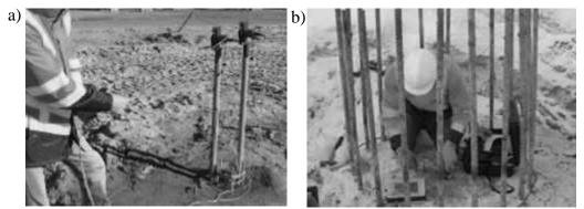
Fig. 1. Methods applied to measure the continuity and length of concrete prefabricated piles [1, 2]: a) Cross-hole Sonic Logging, b) Pile Integrity Test (PIT)
