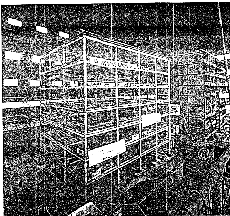
Fig. 1 : The in-situ concrete frame building project at Cardington.
